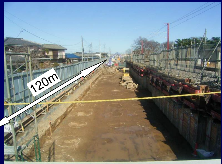
<After the ground improvement>
