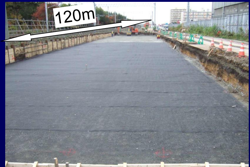
<Arrangement of geogrid >
