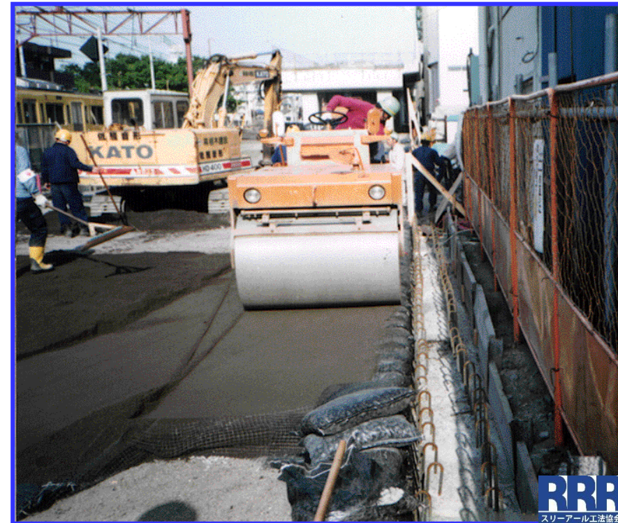
2) Placing geosynthetic & gravel gabions
