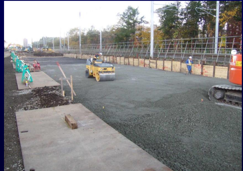
< Construction of the slab >
