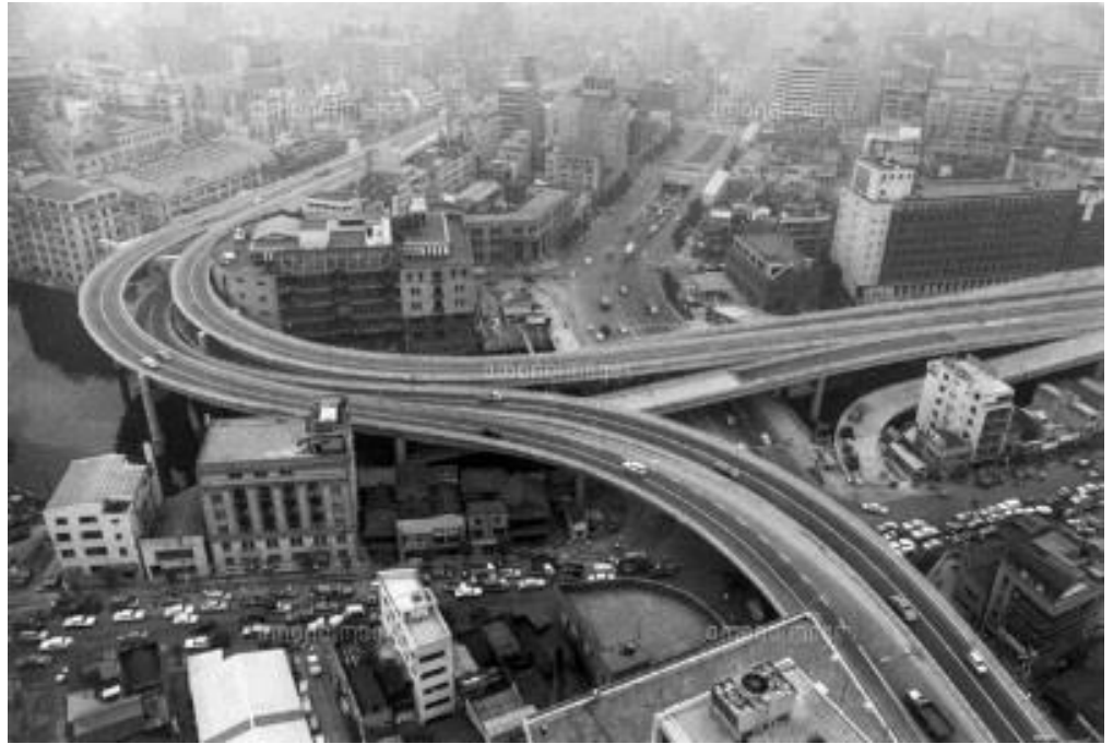
<Metropolitan Expressway, Tokyo> 7
