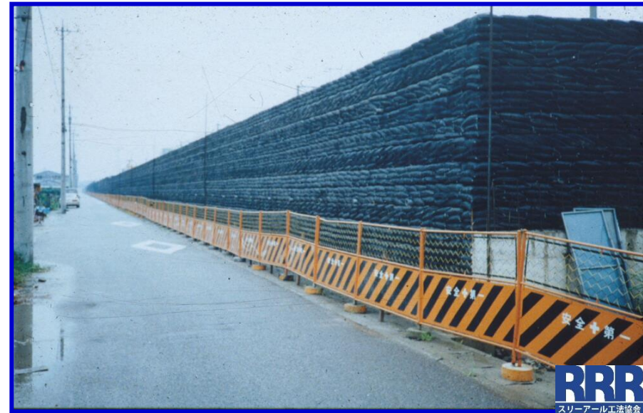
2) Placing geosynthetic & gravel gabions
