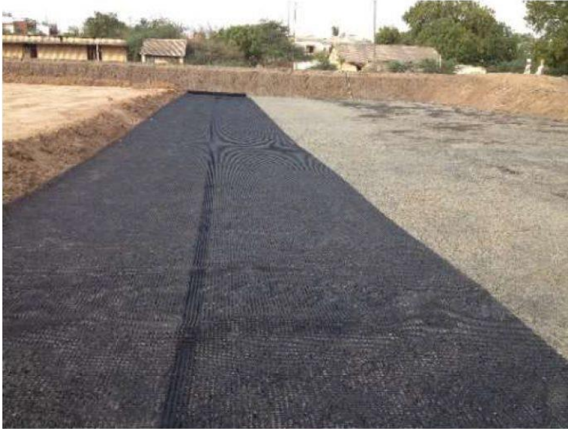
Arrangement of geogrid in CGS improvement layer
