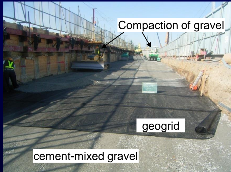
<Construction of the slab, 2009/4>
